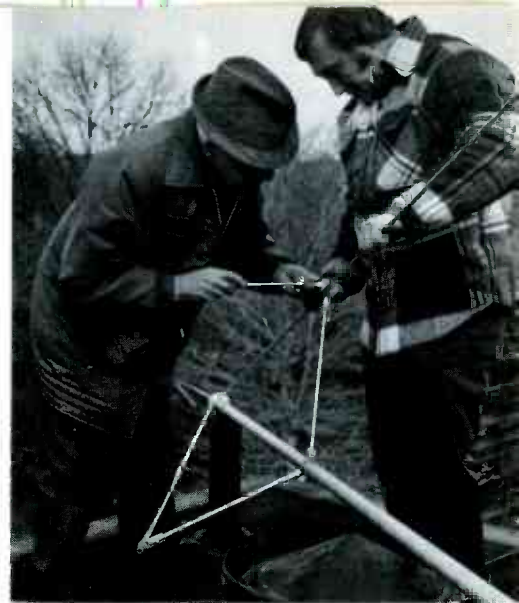
Base station work includes the assembly and erection of the antenna.
